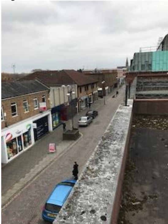
View from the roof looking down the High Street towards Jubilee Walk
